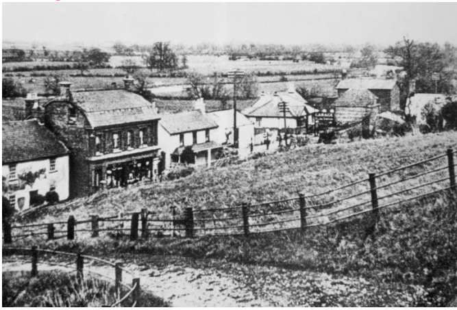
the original cart track to the 'down' platform
